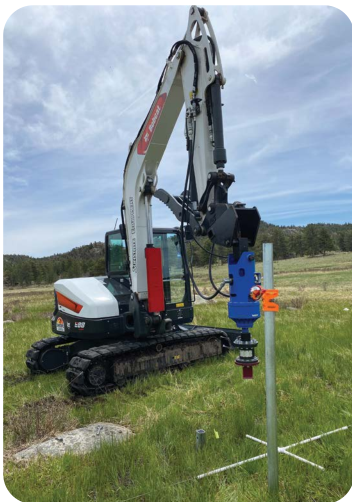
Project Manager Kaleigh Keohane uses an excavator with blue auger attachment and level to drill helical piles (huge screws that provide the foundation for the concrete path).
