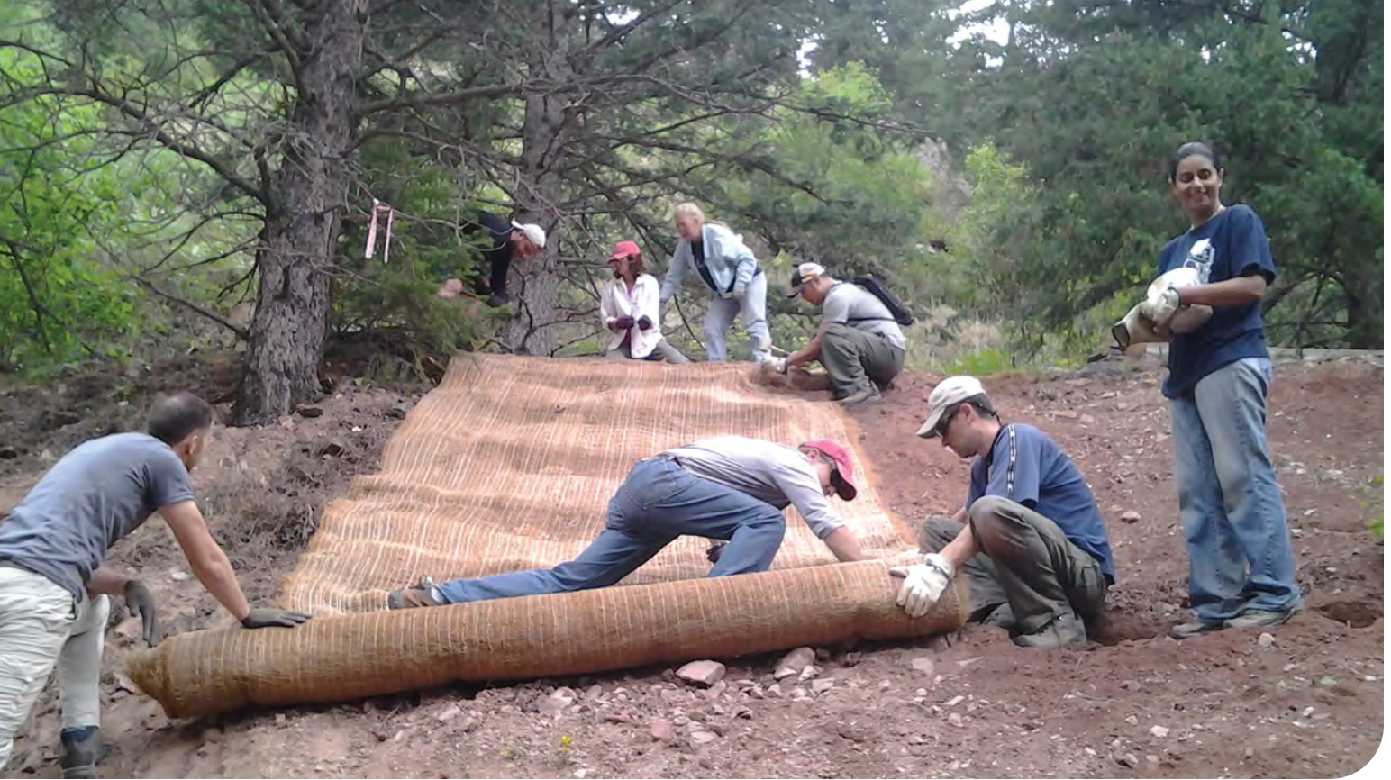
Volunteers lay down a biodegradable mat to control erosion and allow native seeds time to grow after the flood damaged Eldorado Canyon, 2014. Gifts like yours help WRV spring into action long before emergency funding becomes available. 2014 photo.
