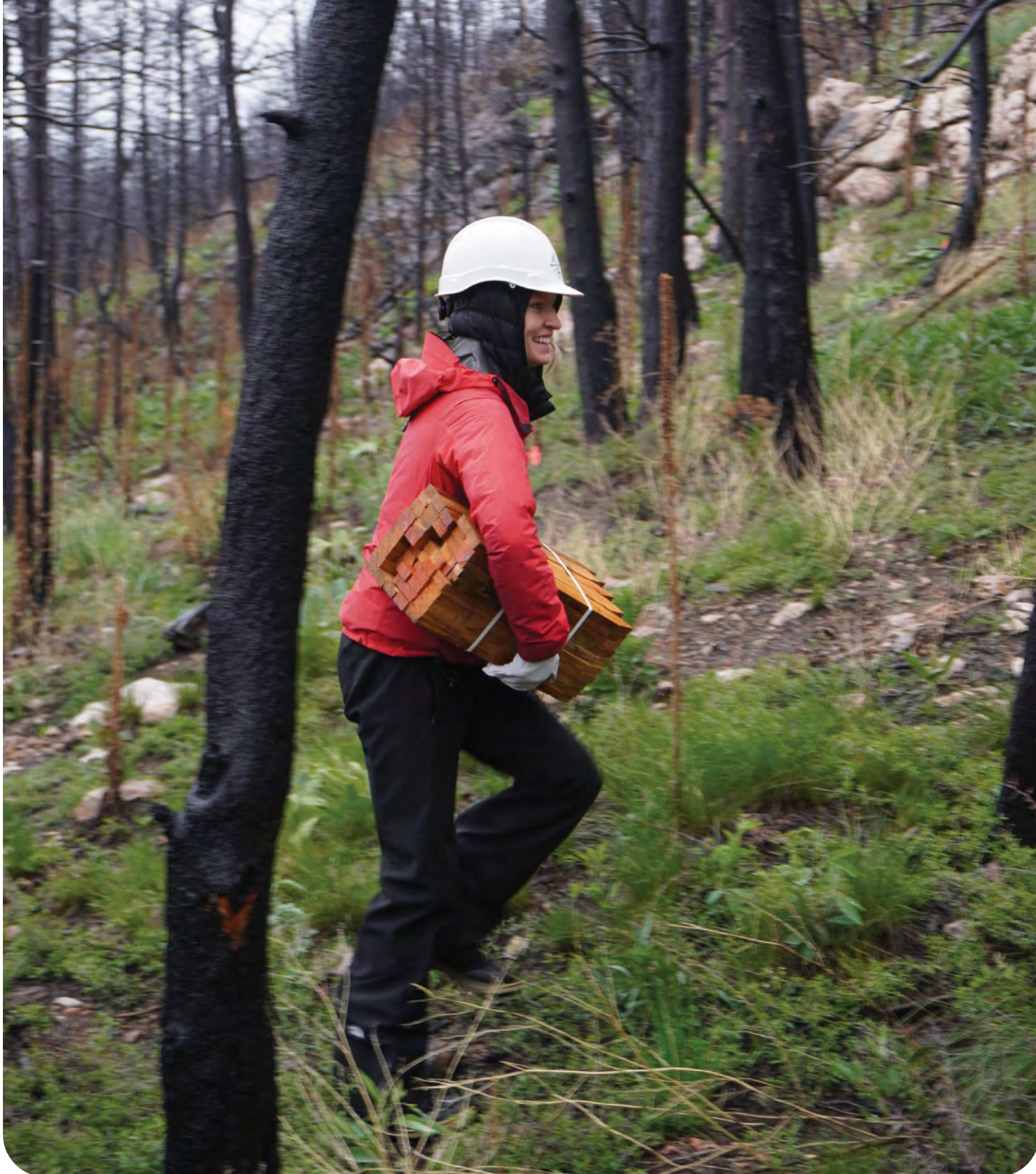
A volunteer carries wooden stakes up a slope to hammer into the ground, 2023. These will hold straw wattles in place in the Cal Wood burn scar. Straw wattles slow runoff and capture debris to prevent post-fire mudslides and flooding.
