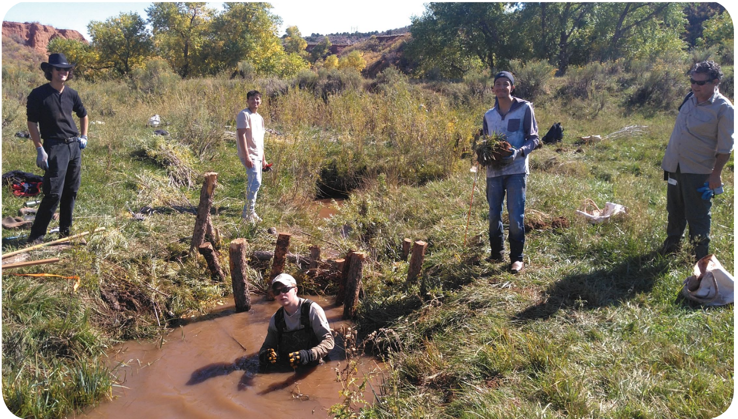
CSU volunteers stand in/next to a stream in Campbell Valley, north of Fort Collins, where they built a beaver-mimicking structure to stop and slow erosion and improve water quality. Your gift supplied the tools, trained leaders, and direction. WRV Board member and Crew Leader, Pedro Lopez stands at right. WRV photo, 2022.
