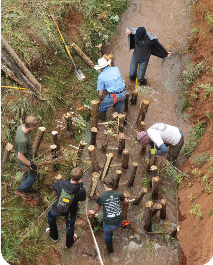
Support from donors like you allowed WRV's staff to partner with colleges and universities in projects like this. Rick and the students drive logs into the stream bank in Campbell Valley to create an "induced meander". Structures like these slow and clean the water and nourish streamside plants. Rick Knight photo, 2016.
